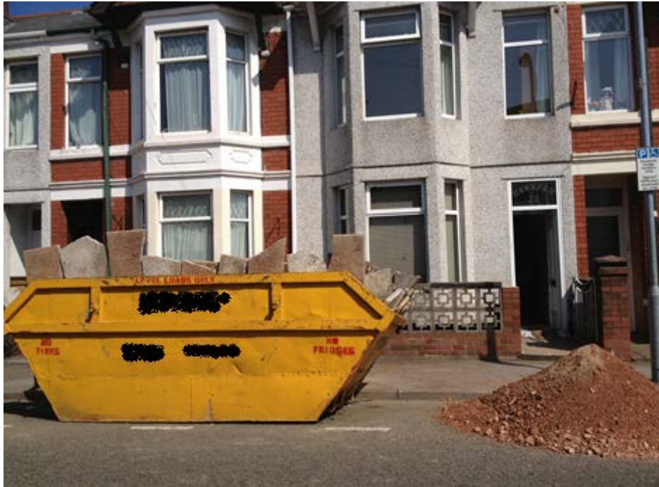
Example of Highway Obstructions
